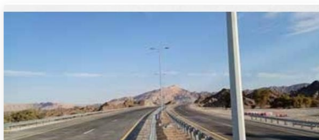
Construction of Balance Works for Dualization of Mahdha-Al Rawdha Road
