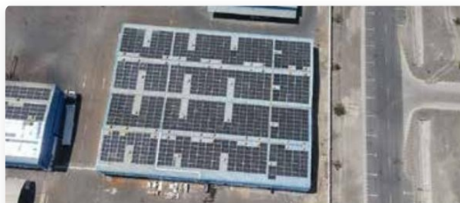
683 kWp On-Grid Rooftop Solar PV Project, Samail Industrial Area
