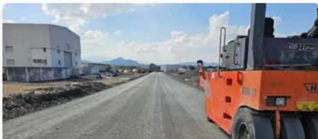
Construction of Internal Road at Misfah, Phase-1 — 17.8 km
