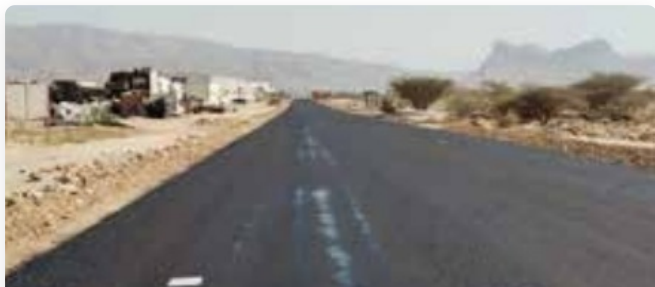
PDO Projects in road construction using Foam Bitumen & Asphalt
