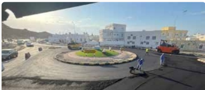
Rehabilitation and development of roads in the Wilayat of Sur
