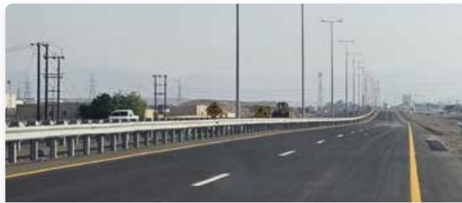
Design & Construction of Dualization of Road, 14.43 km — Khaburah R/A to Batinah Expressway
